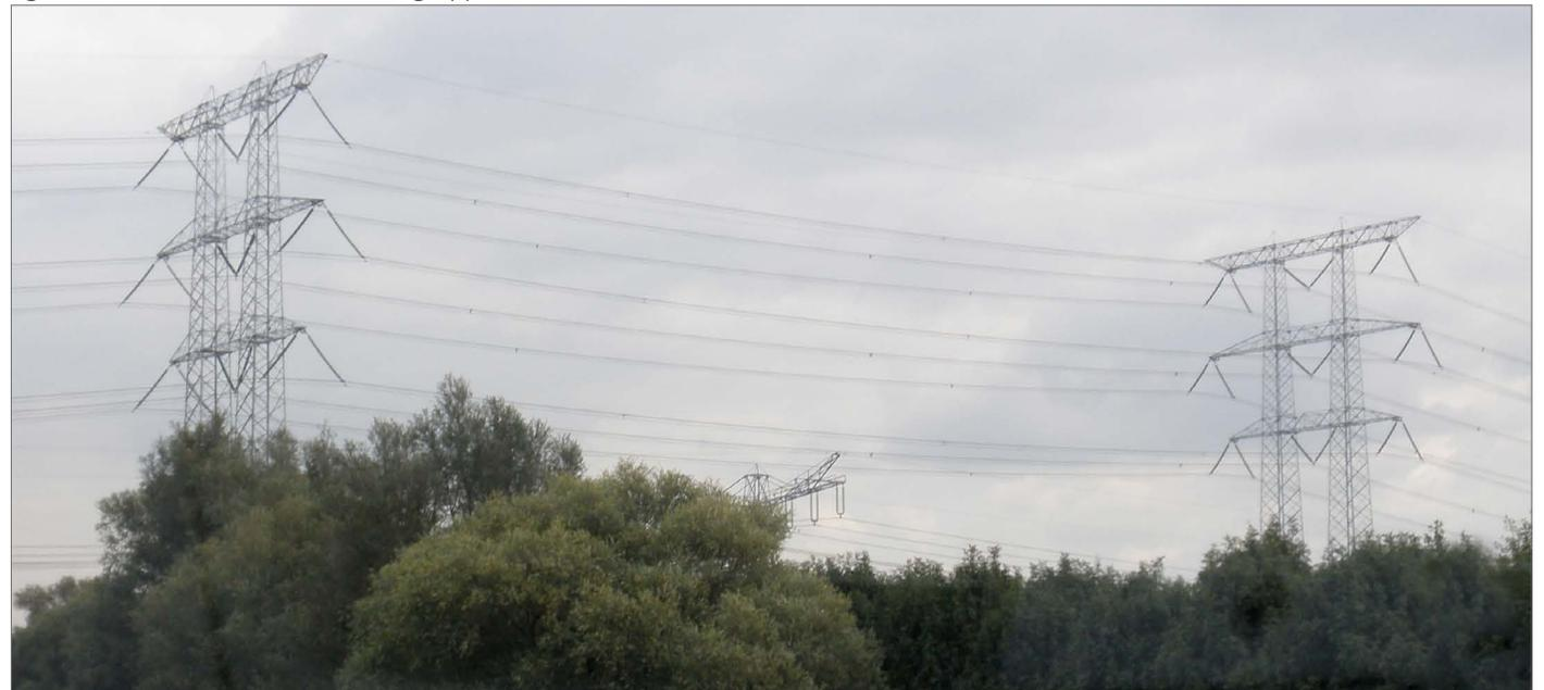
suspension of the conductors also has a different shape. For instance, in case of a lattice pylon the insulators will hang horizontally as opposed to the insulators at a support pylon that hang vertically. The result is that a pull pylon is lower than a support pylon.
