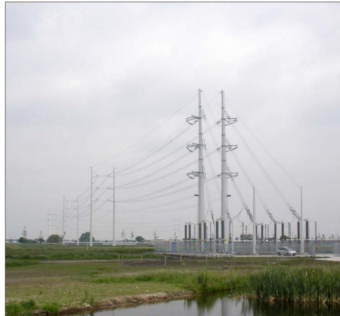
fig. 30 a *transition point bipole pylon 150+380kV (Project 2006-2016)*
