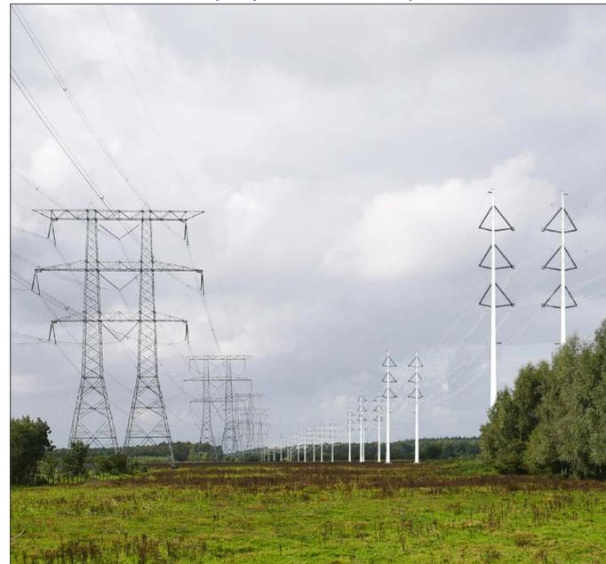
fig. 50 Different forms of possible bundling of existing overhead lines (left) with new ones (right) to gain insight into the effects on grid level and line level (Project 2015-2022)
