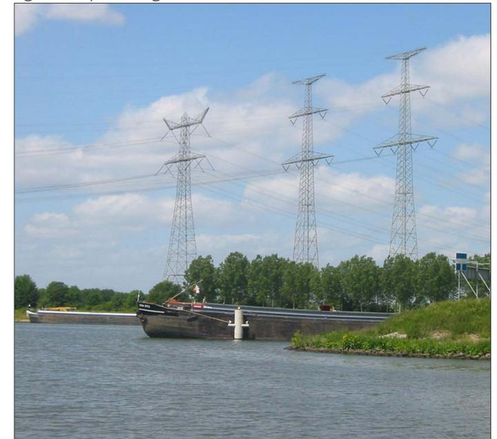
For example, when crossing a dike with a road, a river that is navigated by large vessels, or a building. In such a situation a choice for higher pylons is sometimes made in combination with a shorter field length. High pylons strongly determine the appearance of a line. It is important that a visual recognizable connection is created between the high pylons and the reason for them in the landscape.
