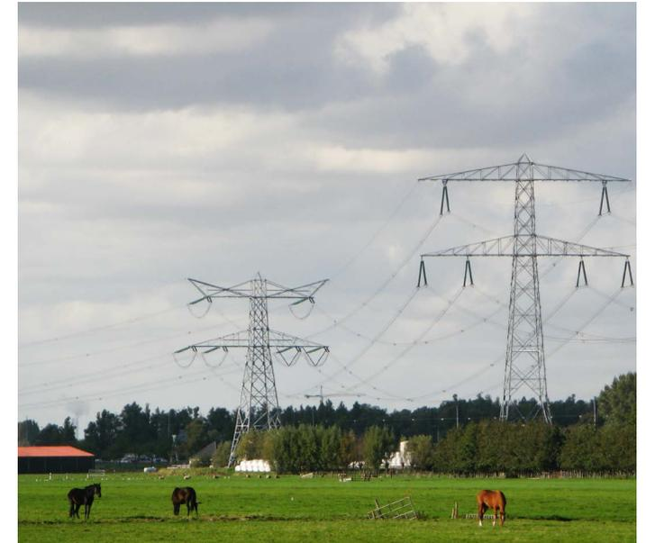
fig. 27 b *Corner lattice pylon with different design, wider and heavier; insulators are horizontal so the pylon is lower*
