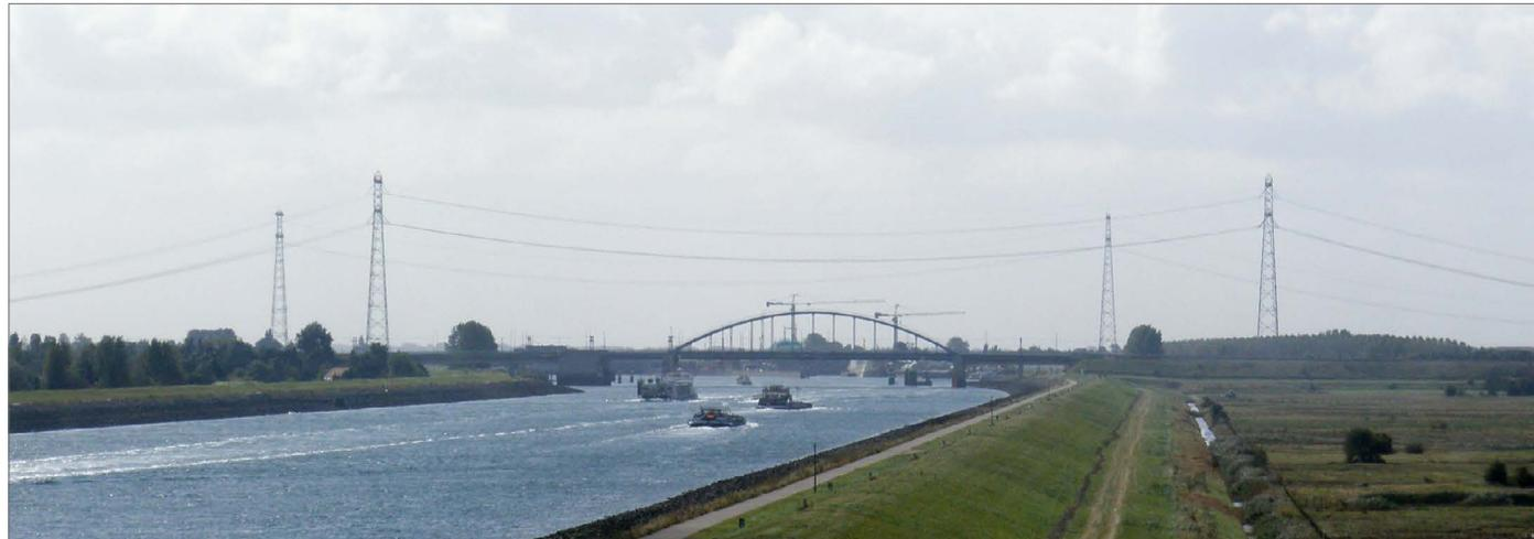
clearer than when you stand at a distance and look more or less at right angles toward the overhead line. Sometimes it might be better to divide a sharp 40 degree angle into a few less sharp angles, so that the optical difference between the pylons changes step by step.
