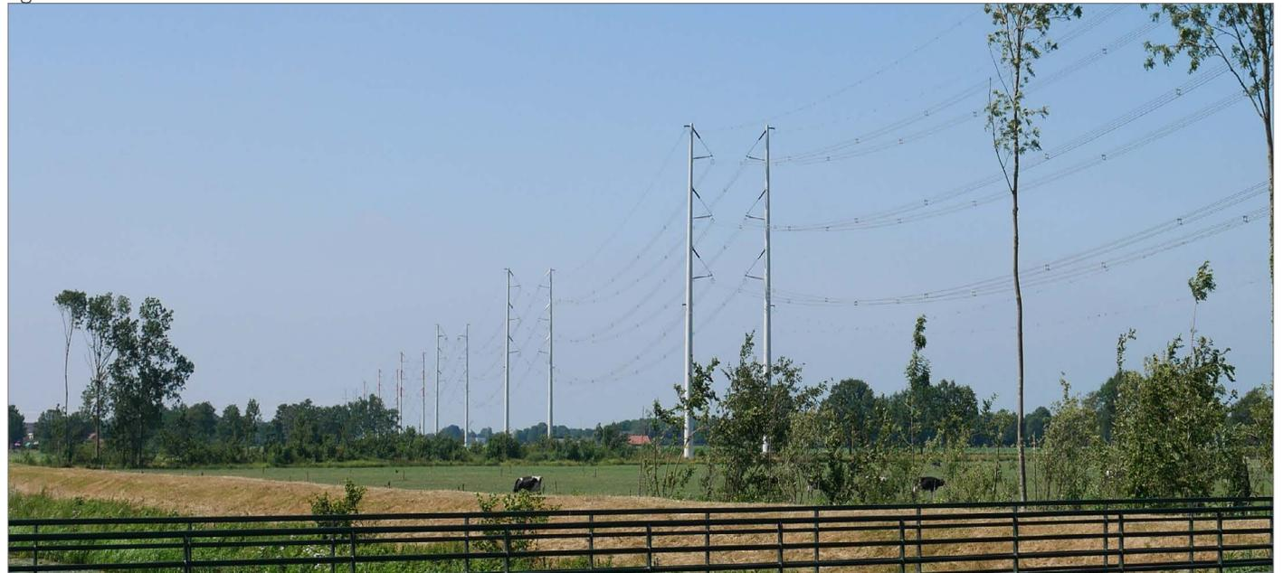
Basic design principle, "a straight line is the shortest connection between two points", already stated in the study by Vrijlandt (Vrijlandt et al., 1980). It is under all circumstances most beautiful solution because it reflects the main function of electricity transport in the most efficient and effective way. However in most situations it is not possible to make a straight line.
